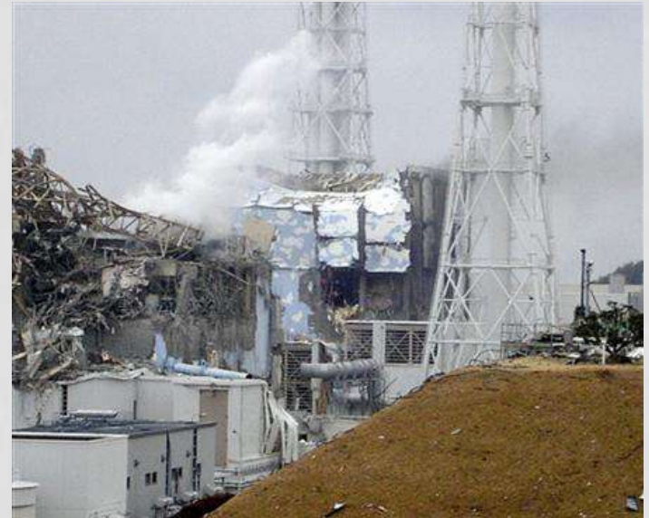
Reactors on 15 March
