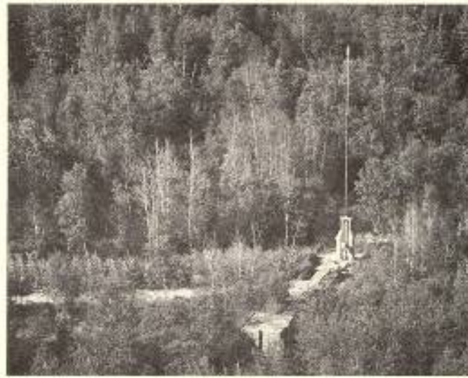
FIGURE 2. FIG irradiation tower, photographed in 1973, showing the 10 m screen, tower supports, base equipment, service road, and wood burned tower.
